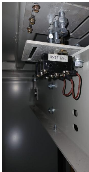
Pasang sensor Seismic, Pasang Sensor Over Load, Full Load, Light Load
